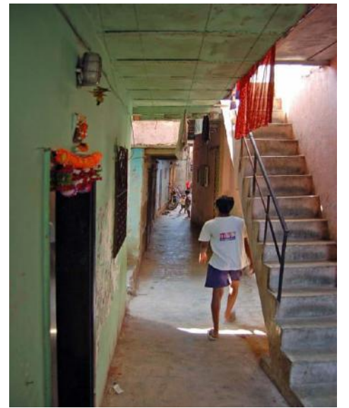
Fig 6: Absence of handrails
