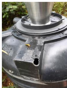
(b) Hole for inserting pipe
