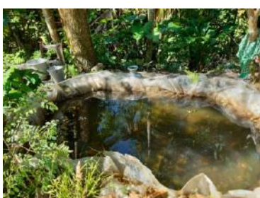
(d) Plastic coated soil embedded water reservoir
