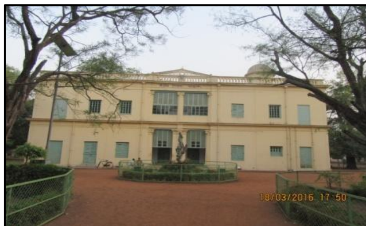
Plate-2: Santiniketan Bari (first building at Santiniketan)
